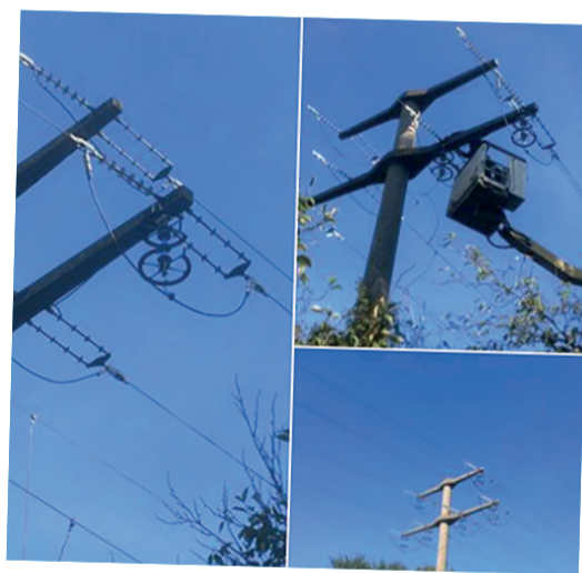
First Streamer installation in Germany (Westnetz): innovative lightning protection solution - SAd35z. News comes later...
